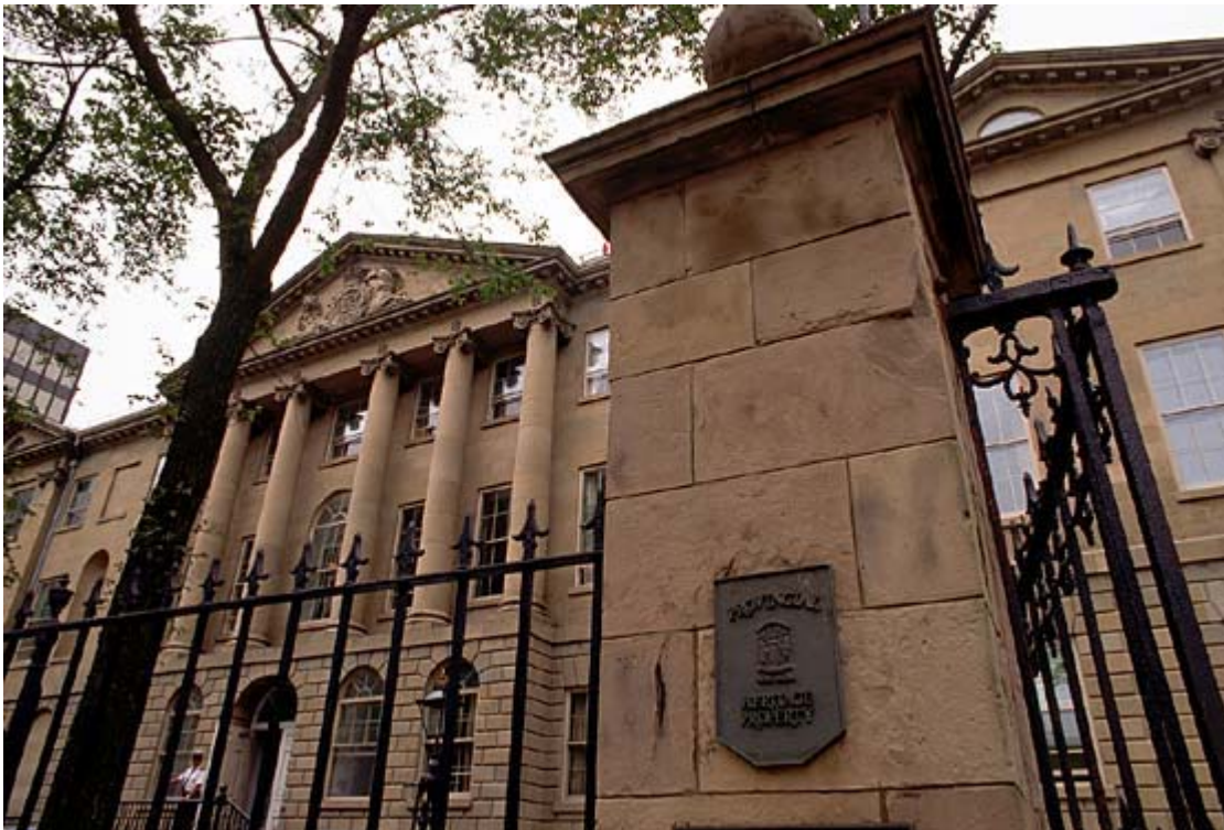
Province House (1811-1819), in Halifax, Nova Scotia, draws inspiration from the Neo-Classical style promoted in Britain by architect Robert Adam. Among the Classical details of this Canadian building, where the Nova Scotia parliament meets, are Ionic columns topped by a triangular pediment, resembling the front of a Greek temple.
